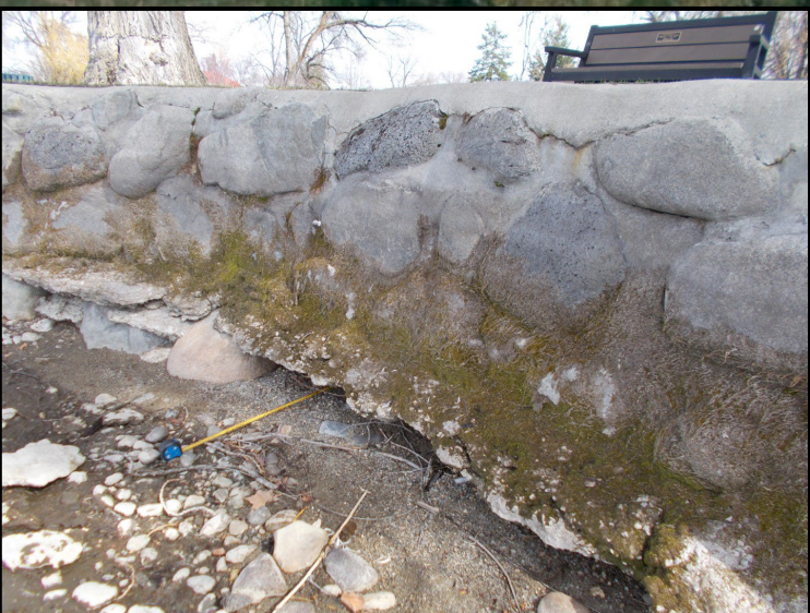
Vertical scour at base of wall post flood
